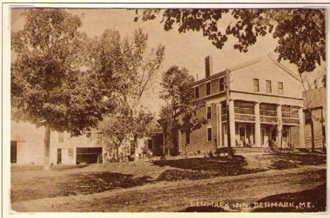
Denmark . Oxford County . Maine . Ca. 1910.
